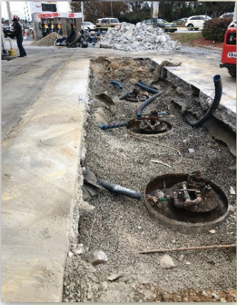
Exposed Tank Field with old flexible fuel piping removed
