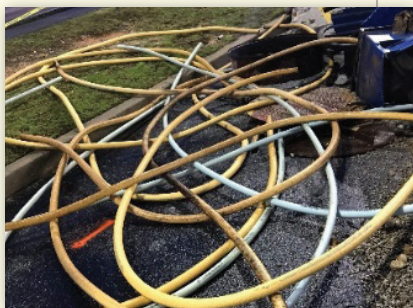
Removed Failed Flexible Fuel Piping
