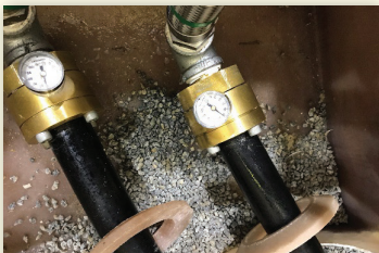
DoubleTrac ® running through new UDCs
