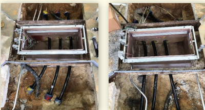
DoubleTrac ® running through new UDCs
