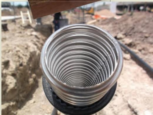
*The double wall construction is dimensionally stable and will not “grow” due to exposure to fuel.*
