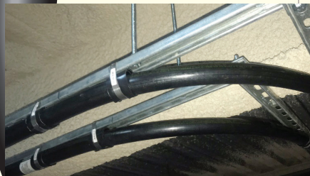
Flexibility of 1" DoubleTrac® (12" minimum bend radius)
