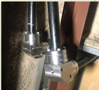
DoubleTrac 90 Degree fittings that allows for continuous interstitial communication. (NO BY-PASS HOSES NEEDED)
