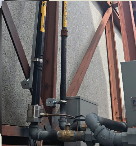
DoubleTrac piping supply and return line to day-tank
