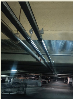
Parking garage (1" DoubleTrac long continuous piping runs).
