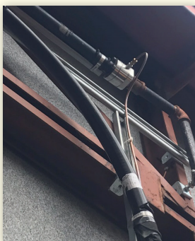
Day tank return line secondary containment continuous monitoring
