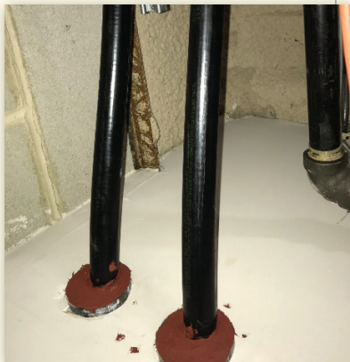
Mechanical Room Floor penetration (4" Casing filled with Fire Caulk)
