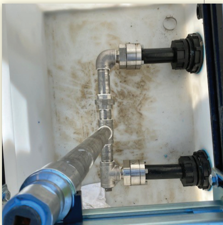
1-1/2" DoubleTrac® entering and exiting the UDC (Under Dispenser Containment Sump).
