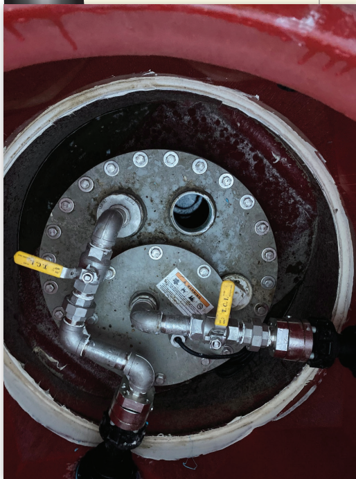
1-1/2" DoubleTrac® exiting and returning to Underground Storage Tank.
