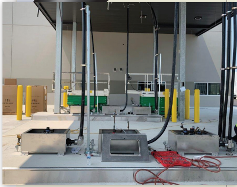
2" DoubleTrac® piping with 90° Elbows for Off-road Diesel dispenser (Left) and Master/Satellite Diesel Dispenser (Right) and 1" DEF-Trac® for DEF Dispenser (Center)
