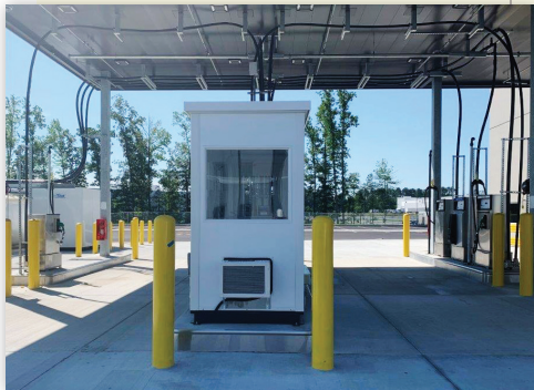
2" DoubleTrac® and 1" DEF-Trac® completed aboveground system for commercial trucks.
