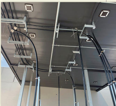
DoubleTrac® with self-contained TEEs for drops and DEF-Trac mounted on the structure below the canopy deck.
