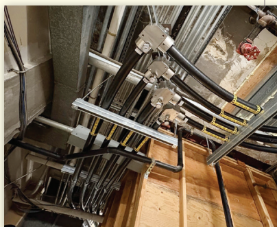
2" DoubleTrac® Dual Fuel Oil Supply (FOS) and Fuel Oil Return (FOR) sweep 90 to double-wall stainless elbows.
