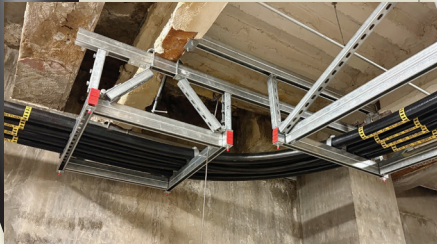
2" DoubleTrac® Dual Fuel Oil Supply (FOS) and Fuel Oil Return (FOR) sweep 90.
