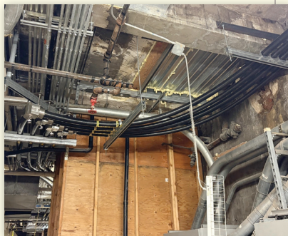
2" DoubleTrac® Dual Fuel Oil Supply (FOS) and Fuel Oil Return (FOR) sweep 90 to double-wall stainless elbows.
