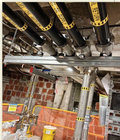
2" DoubleTrac® Dual Fuel Oil Supply (FOS) and Fuel Oil Return (FOR) sweep 90.
