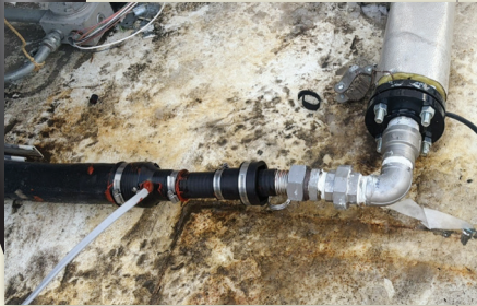
DEF-Trac® piping Connection at the aboveground storage tank outside.
