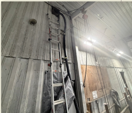
DEF-Trac ® piping second wall penetration and sweeping turn down to the dispenser.
