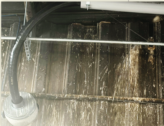
DEF-Trac ® piping third sweeping turn and second wall penetration.
